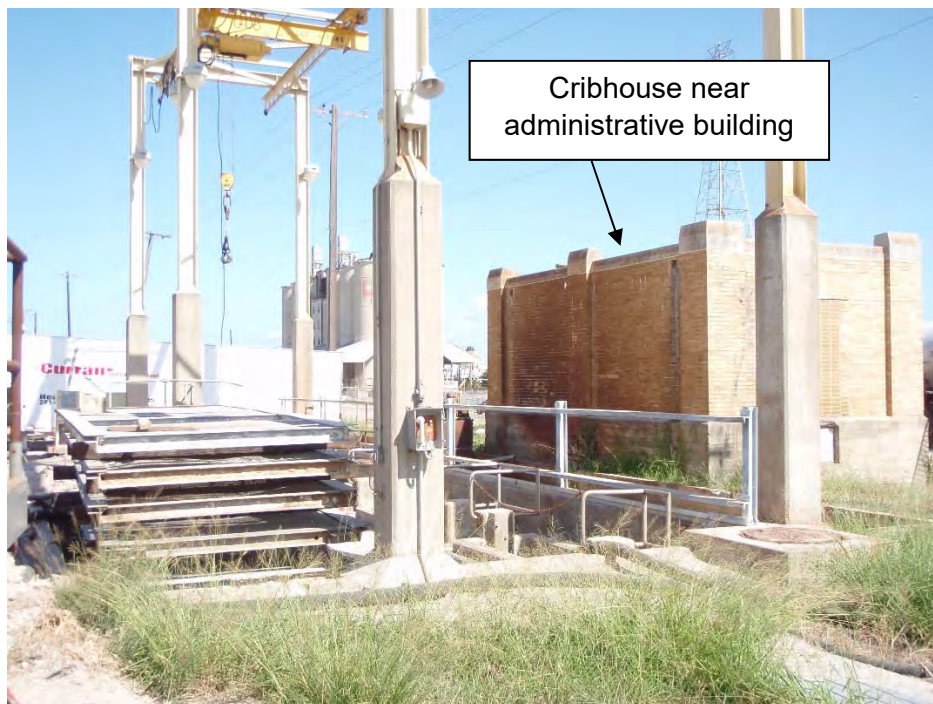
2. Cribhouse near administrative building.
