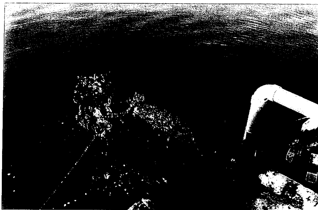
Figure 7. Fouling by Oysters of the Head Box of the Inner Harbor Intake Pipe
